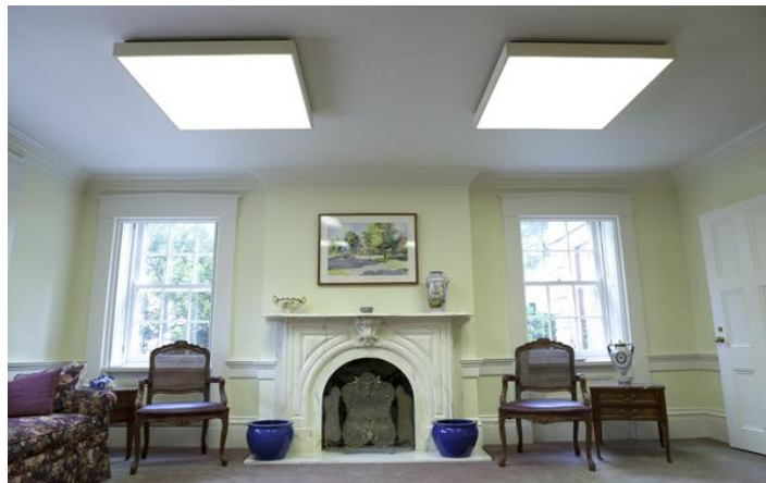
Borealis T8 LED Tube Lighting Installation
